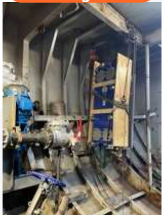
Heat recovery & bilge
